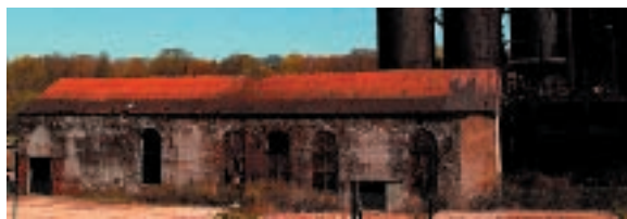
Original Foundry, Bethlehem, PA
