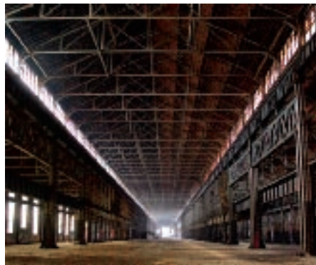
No. 2 Machine Shop—Interior
