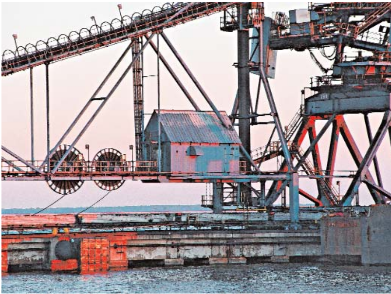
above left Loader Detail (Sunset) —Dominion Terminal Associates, 2005 Digital Print H. 28" L. 38" (unframed) Edition: 5
